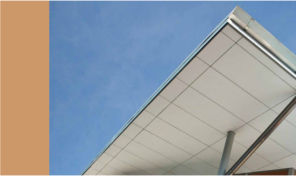
CLG EXTERNAL FC SOFFIT, PAINTED. EXPRESSED JOINTS
