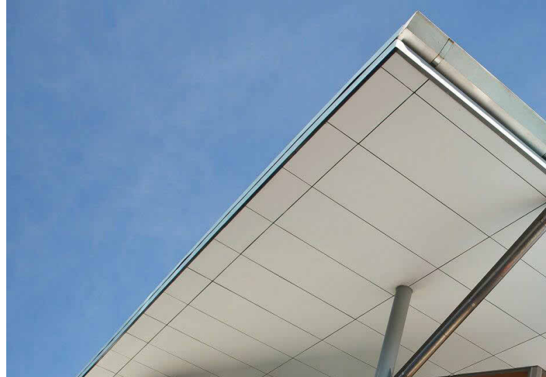
CLG EXTERNAL FC SOFFIT, PAINTED. EXPRESSED JOINTS
